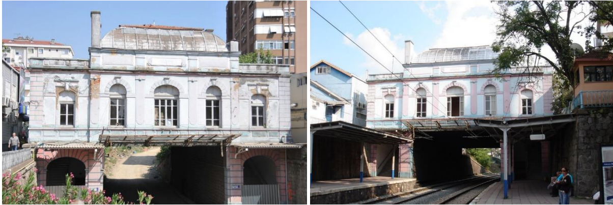
Figure 8. Recent Photographs of the Station Before Strengthening
